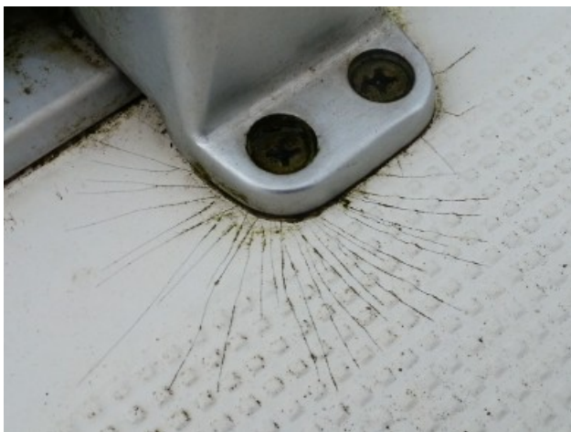
Cracks in the gel coat
